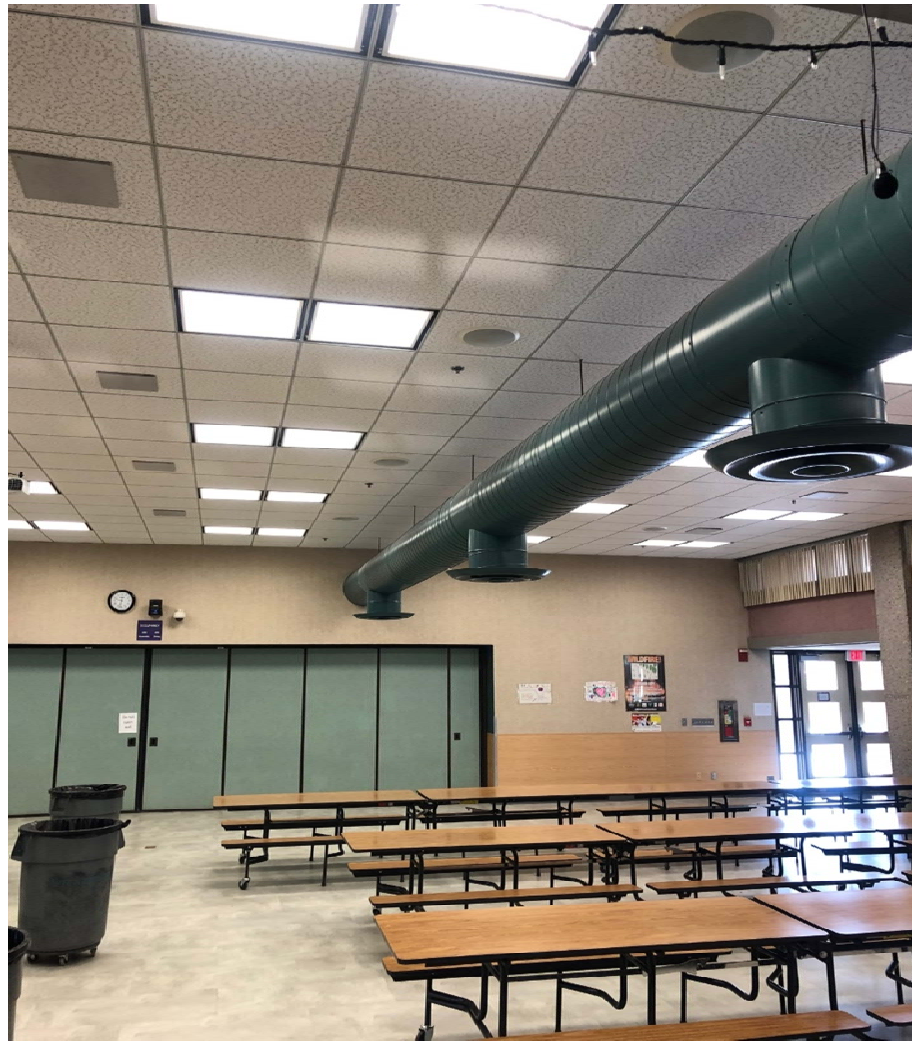
Water Remediation, T-Bar, Lighting Multi-Purpose Room - Gateway
